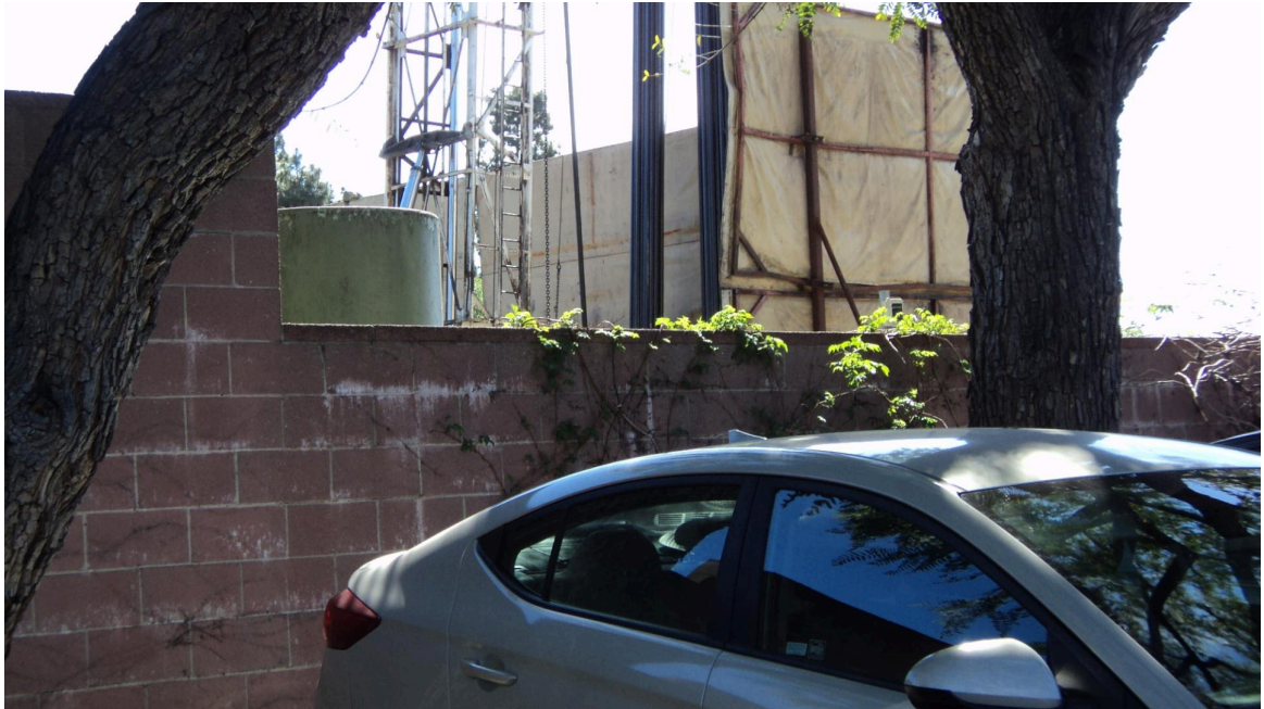
Looking Southeast. Workover rig performing unspecified work. West facing soundmat does not fully cover the operation being performed. (Photo taken March 13, 2026)
