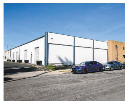
A BUILDING at 13871 West St. in Garden Grove is being converted into the Central Cities Navigation Center, which is expected to be operational in June 2024.
