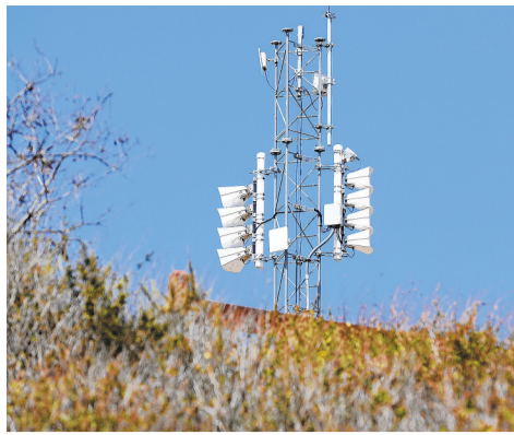
A SET OF speakers for the outdoor emergency warning system at Alta Laguna Park in Laguna Beach.
