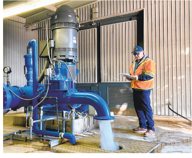
A TECHNICIAN INSPECTS a pump for one of four wells in Fountain Valley that supply 75% to 85% of Newport Beach's water.
