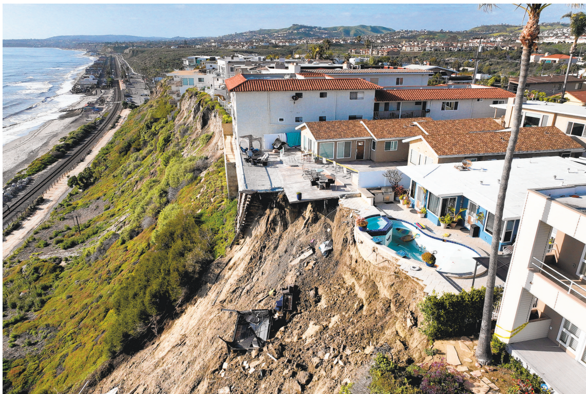
AN AERIAL VIEW of apartment buildings evacuated and red-tagged after heavy rains brought a landslide that left the rear of the buildings in danger of tumbling down the cliff on Buena Vista in San Clemente in March 2023.
