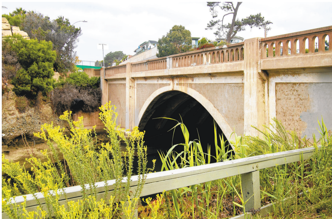
ALISO CREEK Bridge, now renamed Officer Jon Coutchie Memorial Bridge.
