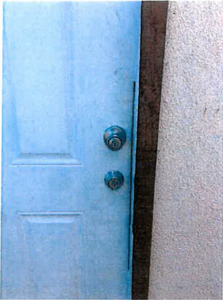
Backdoor 2 nd floor outside
