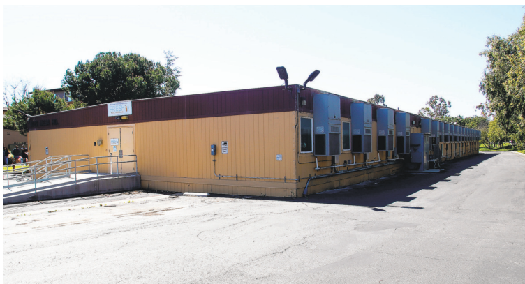
THE AREA for the Mesa Court residence housing expansion at UC Irvine.
