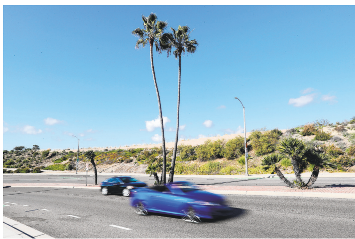
A PEDESTRIAN bridge will be built over Superior Avenue to connect Sunset View and Sunset Ridge parks in Newport Beach.
