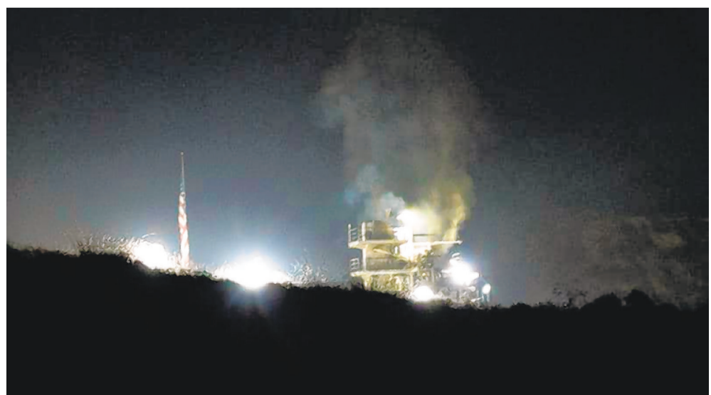
A PHOTO of the All American Asphalt factory in Irvine.
