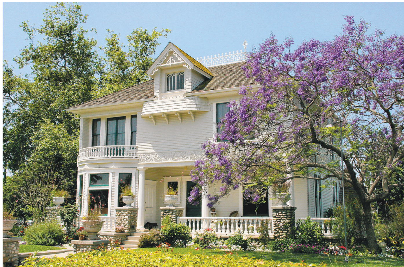
THE HERITAGE MUSEUM of Orange County is raising funds for repairs to the historic Kellogg House's roof.
