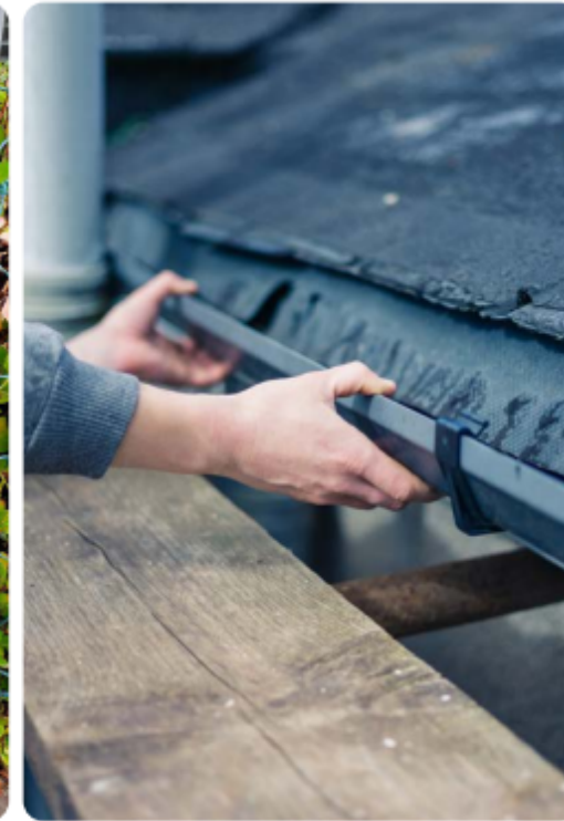
Rain Gutter Replacements
