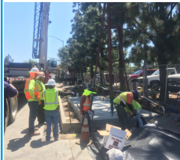
Alamo Salvation Council District 9 Construction
