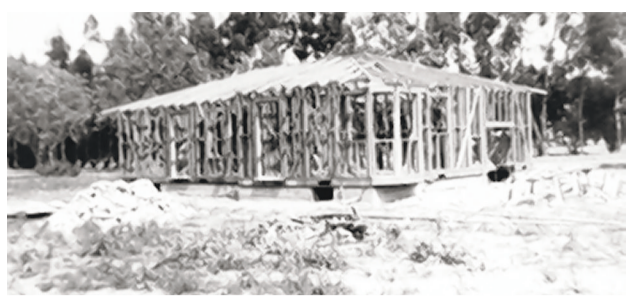
FRAMING THE HOUSE , built on 23rd Street and Orange Avenue on the Beardsley farm.
