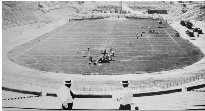
20 Photograph of construction of the South end of Rose Bowl Stadium from the Library of Congress 2 21 22 23 24 25 26
