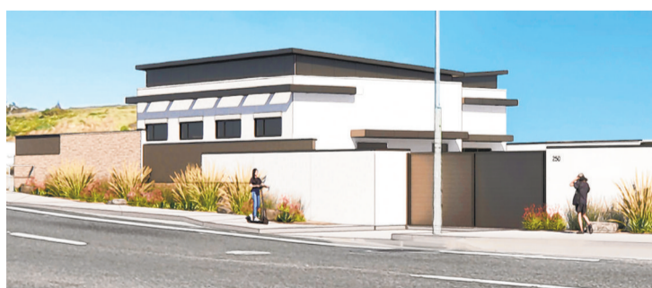
Courtesy of the city of Newport Beach
